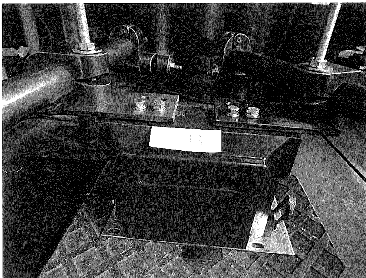
Short circuit test
